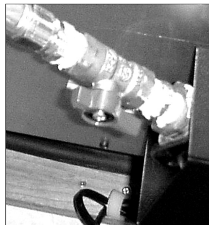
Valve (located under cooktop) shown in OPEN position. cooktop valve.tif
