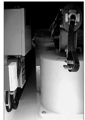
Power Cable Reel.
