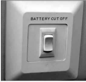
Battery Cut-Off Switch.
