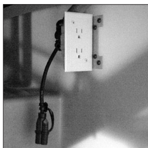
Block heater receptacle located in driver side storage bay.
