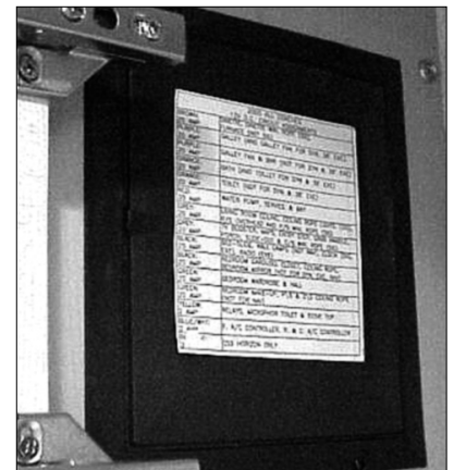
Fuse Panel Label
