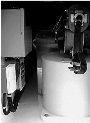
Power Cable Reel
